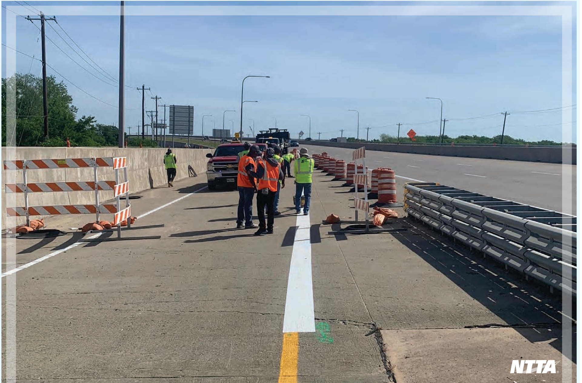
Striping northbound PGA Parkway exit ramp in Frisco
