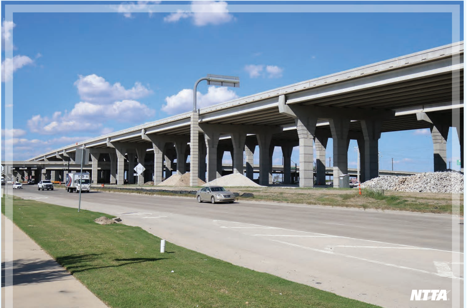
Dallas North Tollway extension bridge over US 380
