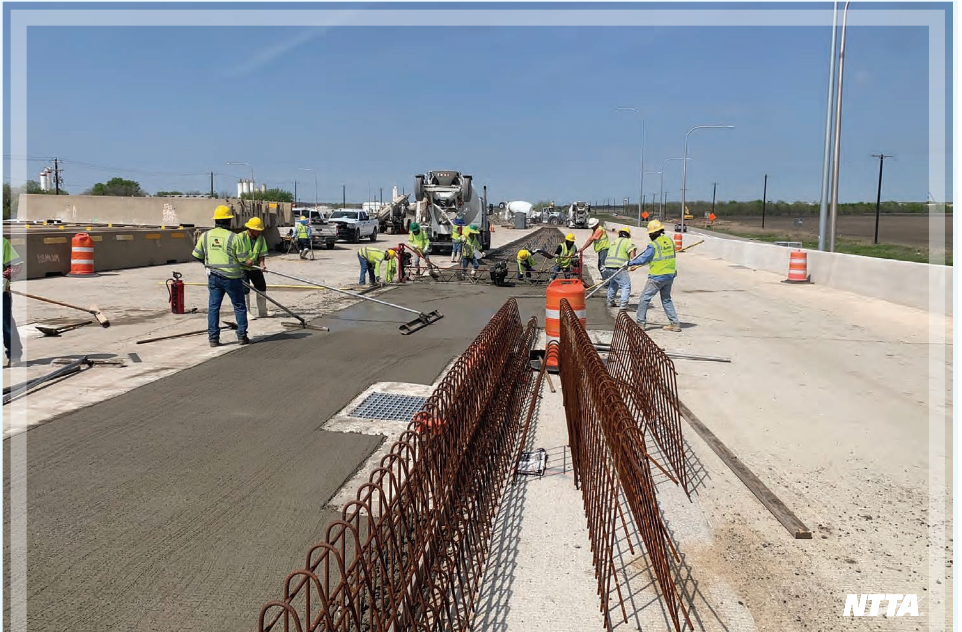
Placing concrete on Dallas North Tollway extension bridge over US 380
