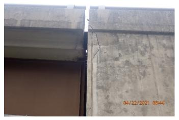
Figure 11: DNT bridge abutment cracking at Harry Hines
