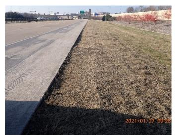
Figure 35: CTP pavement edge drop-off SB at N Oakmont Blvd.
