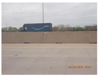
Figure 2: DNT barrier wall spall NBML S of Eldorado Pkwy
