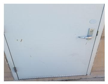
Figure 39: CTP MLG1 rust developing on door
