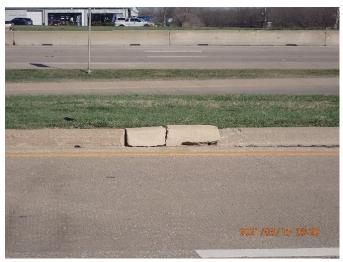
Figure 27: SRT curb damage NB frontage of FM 544
