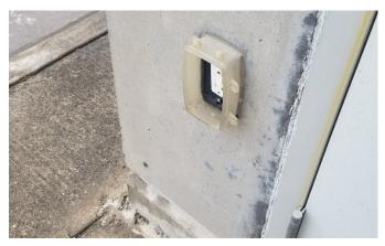
Figure 32: SRT MLG2 – electrical box cover missing
