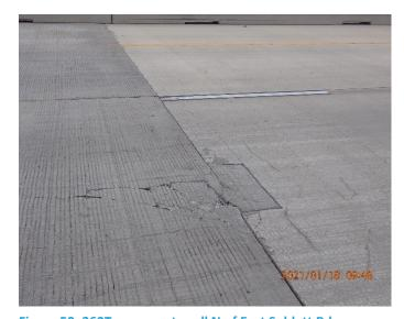
Figure 50: 360T pavement spall N of East Sublett Rd.
