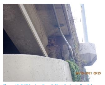
Figure 10: DNT backwall spall SB at Spring Valley Rd.
