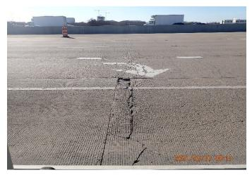
Figure 25: SRT pavement cracking/spalling SB N of Legacy Dr.
