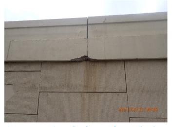
Figure 30: SRT coping spall SB frontage of BNSF Railroad
