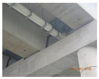
Figure 22: PGBT drainage pipe separation NB bent No. 14
