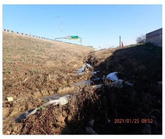
Figure 47: 360T ditch-line erosion at Bowman Branch
