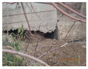
Figure 45: MCLB erosion under abutment riprap West end
