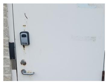
Figure 55: Gleneagles 5900 – rust developing on door
