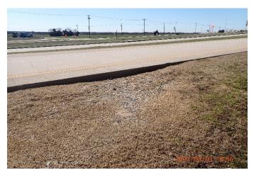
Figure 26: SRT pavement edge drop-off NB exit ramp to Medical Center Dr.
