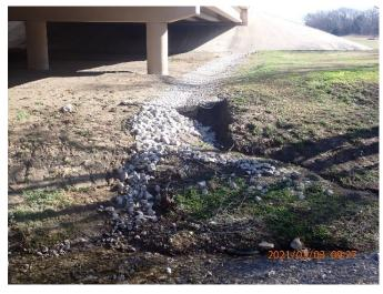
Figure 29: SRT erosion NB at Cotton Wood Creek
