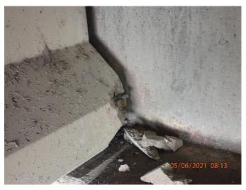
Figure 43: MCLB beam end spall at West abutment
