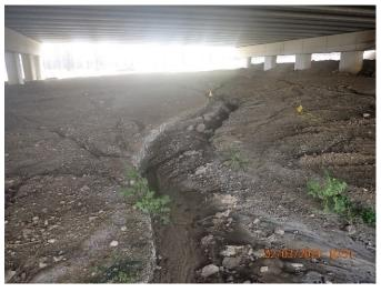
Figure 20: PGBT erosion under bridge S. of Carrier Way
