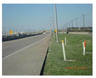
Figure 6: DNT pavement edge drop-off SBML N of Panther Creek.
