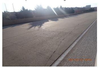
Figure 37: CTP pavement crack S of Arborlawn Dr.
