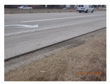
Figure 48: 360T pavement edge drop-off S of Green Oaks Blvd.
