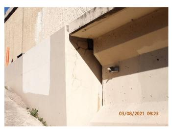
Figure 19: PGBT backwall cracking/spalling at Creek Bridge W. of Preston Rd.
