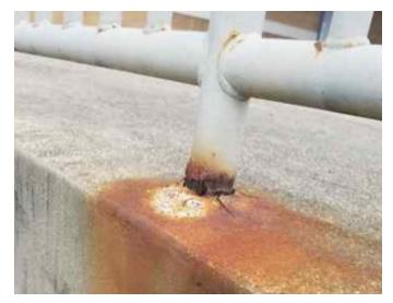
Figure 53: Ohio – rust on railing
