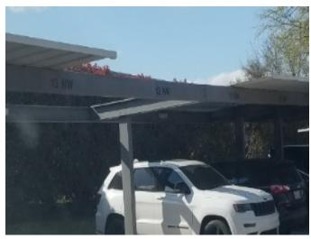
Figure 56: Gleneagles 5900 – canopy roof section missing
