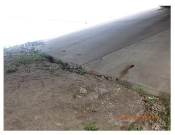
Figure 3: DNT Erosion at Stewart Creek bridge
