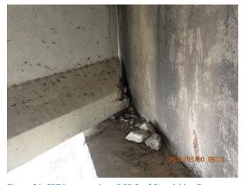
Figure 31: SRT beam end spall SB S. of Standridge Dr.
