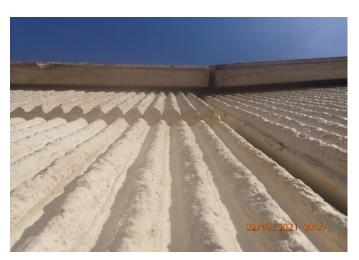
Figure 18: PGBT retaining wall panel movement EB at Egyptian Way
