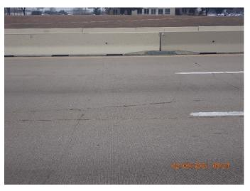
Figure 17: PGBT pavement cracking NB S. of SH 114
