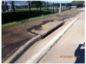
Figure 42: MCLB curb damage at inlet EB West end of bridge
