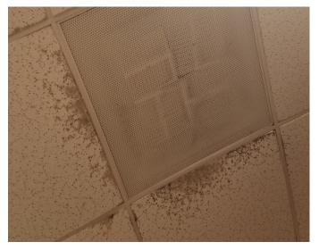
Figure 57: Gleneagles 5910 – water stains on ceiling tiles
