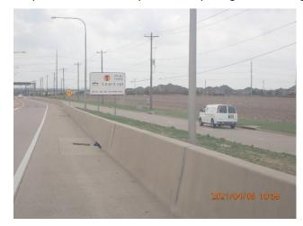
Figure 7: DNT delineation missing on CTB SB ramp at Panther Creek
