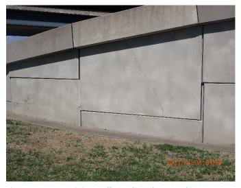
Figure 9: DNT retaining wall panel crack at Panther Creek
