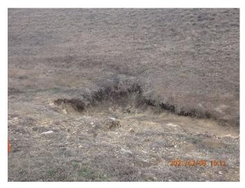
Figure 34: CTP erosion in ditch-line S. of Old Granbury Rd.
