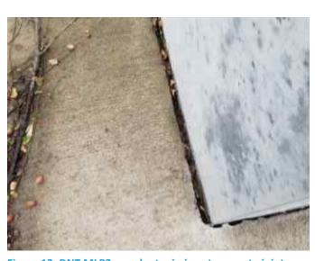
Figure 13: DNT MLP2 – sealant missing at concrete joint
