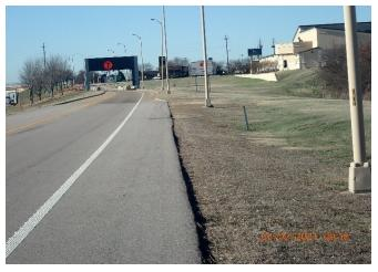
Figure 16: PGBT pavement edge drop-off WB exit to Marsh Ln.
