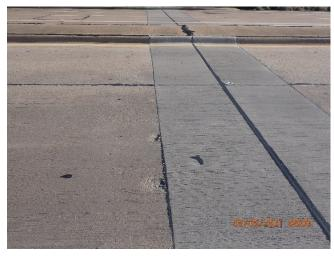
Figure 41: MCLB pavement spall EB West end of bridge
