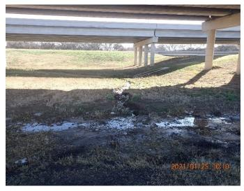
Figure 52: 360T minor erosion under bridge at Walnut Creek
