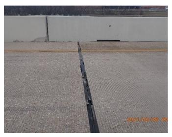
Figure 36: CTP pavement joint seal missing SB at Riparian Woodland
