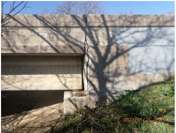
Figure 51: 360T backwall cracking at Walnut Creek bridge
