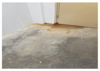
Figure 24: PGBT MLP08 rust developing at door frame
