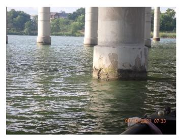
Figure 21: PGBT column spall SB bent No. 41
