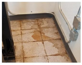
Figure 12: DNT MLP3 – floor damage from water intrusion
