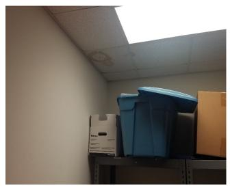
Figure 23: PGBT MLP07 water stain on ceiling
