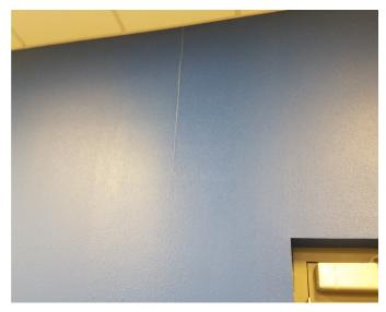
Figure 54: Frisco – crack in drywall
