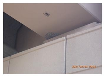
Figure 38: CTP bridge beam spall at Edwards Ranch Rd.
