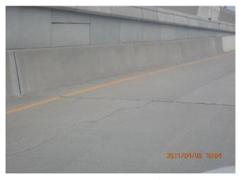
Figure 4: DNT pavement crack on ramp from Main St.
