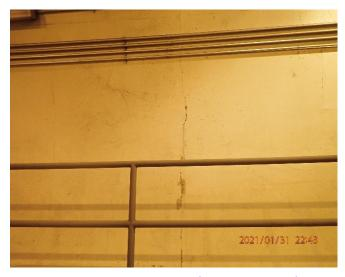
Figure 46: AATT cracking on walls (various locations)
