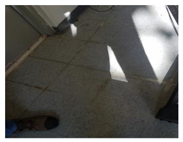
Figure 40: CTP MLG2 SB floor damage due to water intrusion
