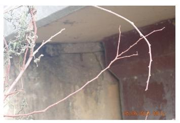
Figure 44: MCLB backwall spalling at West abutment
