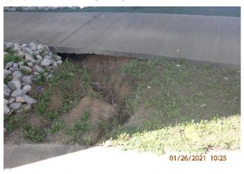
Figure 15: PGBT erosion under sidewalk SB ramp to IH-20
