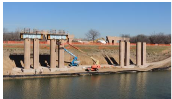
Forming bridge supports on the north side of Trinity River.
