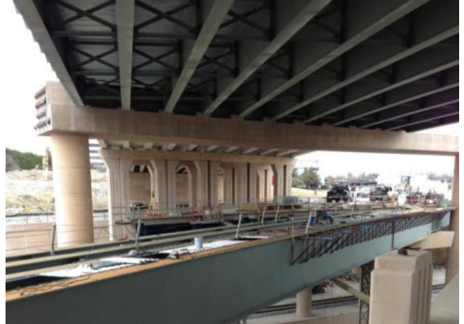
Forming of bridge deck under Hulen Street Bridge.
