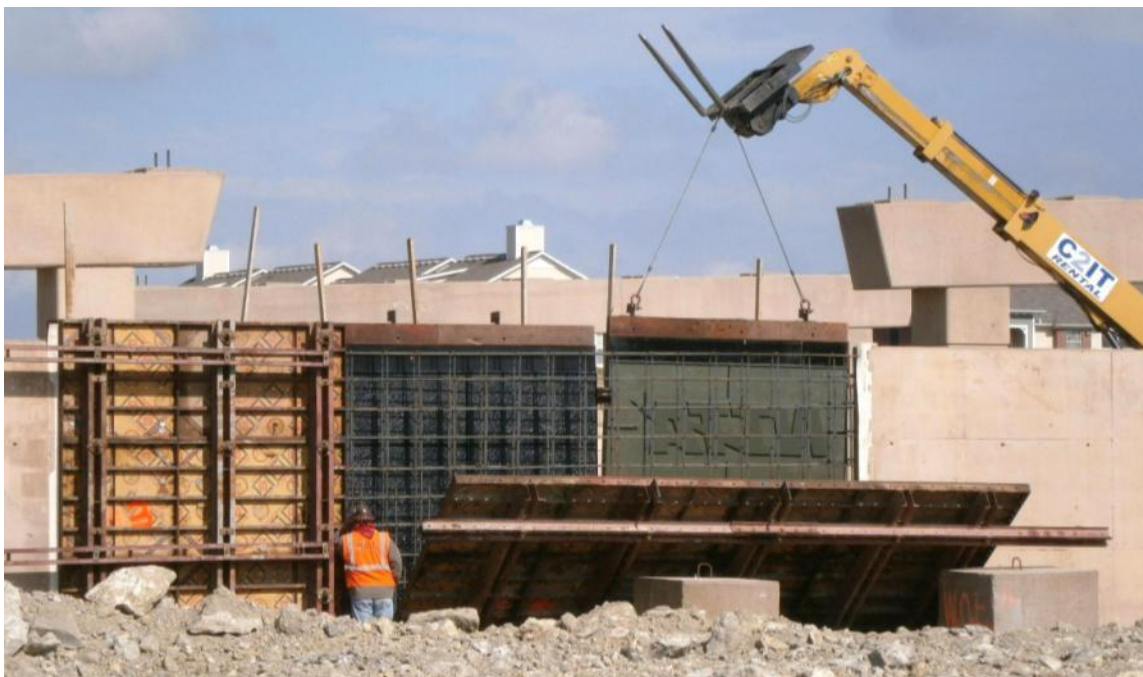
Cast-in-place wall construction on CTP Section 5.
