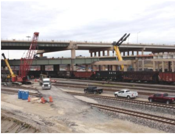
Placing girders for the main lane bridge.
