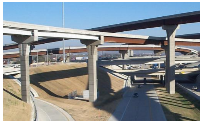
I-30/PGBT Western Extension interchange
