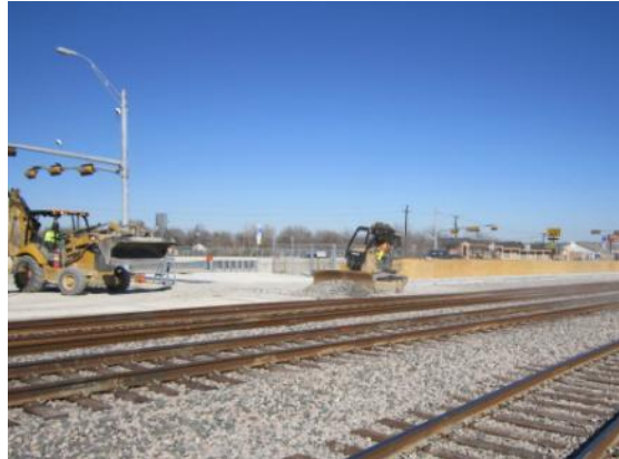
Rail bedding at the UPRR crossing.
