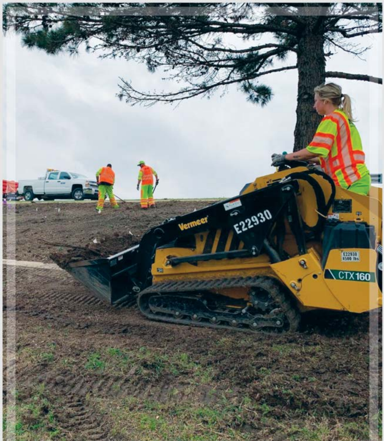
Landscape crew performing erosion repairs
