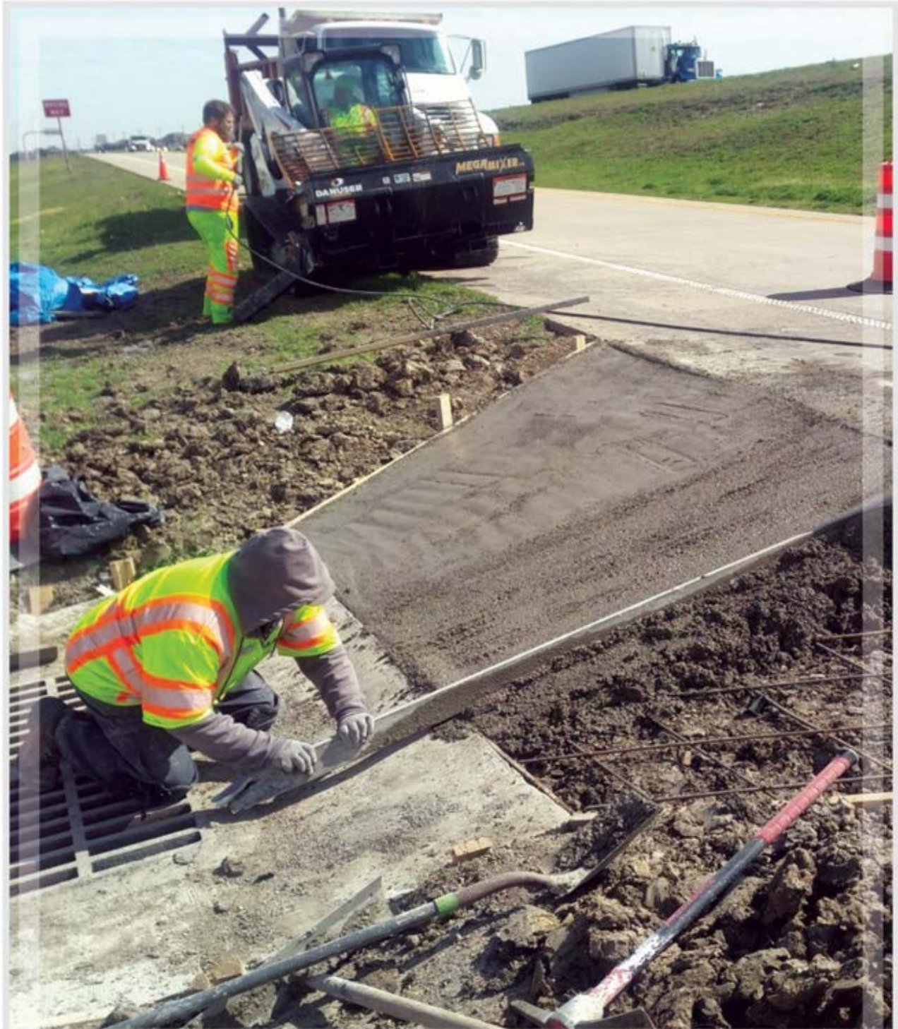
Pouring concrete for inlet drain
