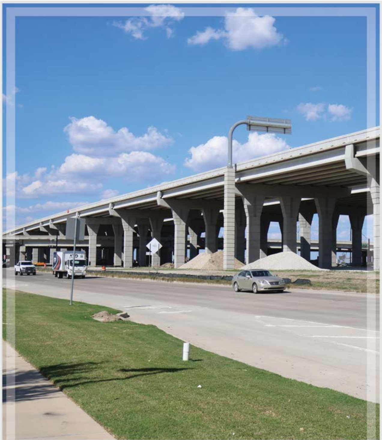
Dallas North Tollway extension bridge over US 380
